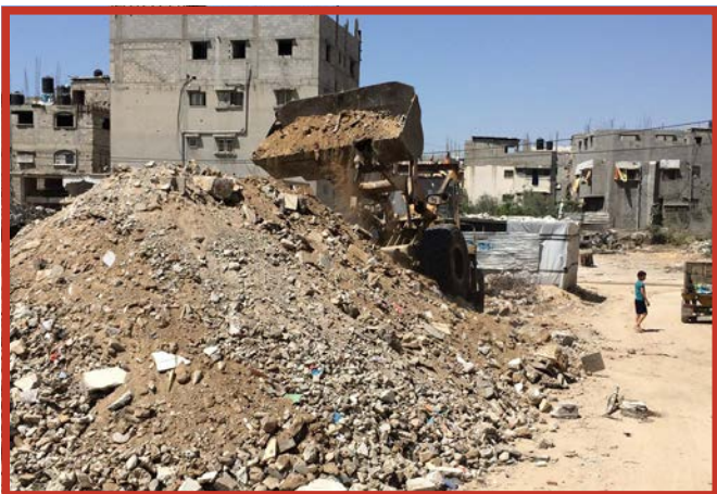
Cleaning rubble in Gaza for rebuilding efforts. Credit: EU/ECHO/Caroline Gluck
